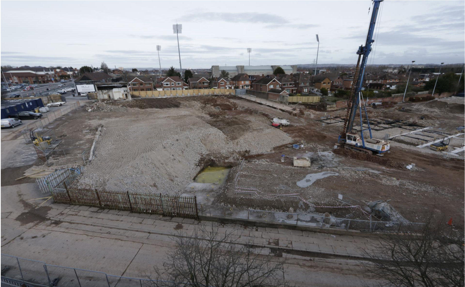
Andersonstown – Works Underway – March 2018
