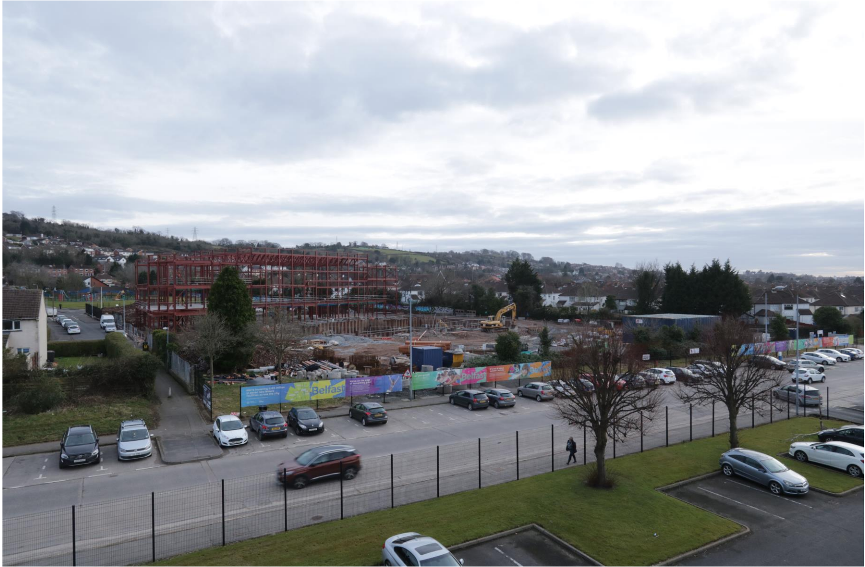
Robinson – Works Underway – March 2018
